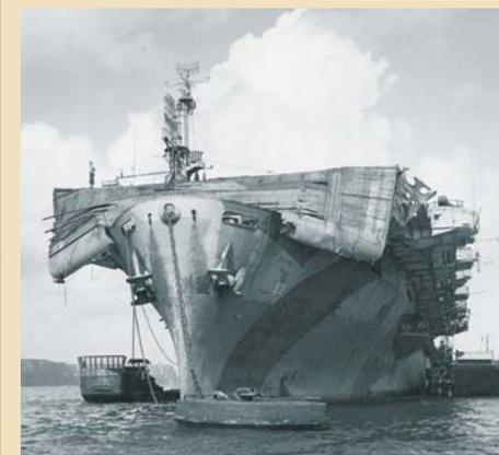
*The power of Hurricane Viper, which struck the U.S. 3<sup>rd</sup> Fleet off Okinawa in June 1945, is evident in this photo of USS Windham Bay (CVE 92).*
